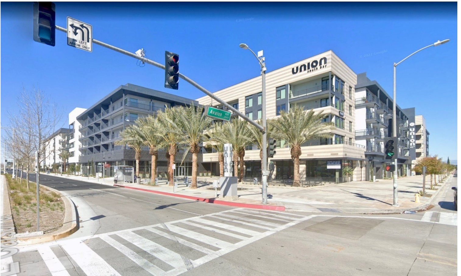
Figure C- I: Union South Bay Photo Example
